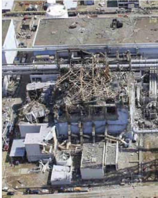
Figure 2: Reactor No. 3 Spent Fuel Pool Area
